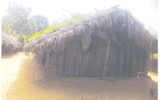
Fig 5.8 : Hut made of bamboo and thatch
